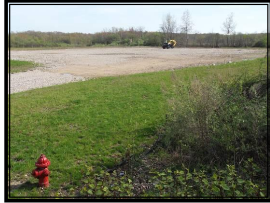
(Looking W from NE corner)
